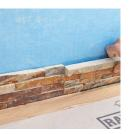
before you apply any adhesive, dry lay out your first row against the wall to help you work out the look you want. Lay them in a brick pattern to make panel joints less visible.
