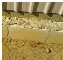
Now fill the joints with mortar using a trowel. Making sure to remove any excess mortar off the face of the wall, to ensure you end up with a clean finish. For any subsequent courses place mortar on top, then apply the next layer of blocks.
