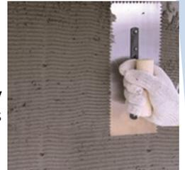
Take your trowel and spread the first course of adhesive at the bottom of the wall. Apply enough for the first couple of rows of stacked stone.
