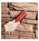
Protect the installation by avoiding cleaning or exposure to rain for a minimum of 7 days. For interior installations, either a penetrating or tropical sealer can be used. For exterior installation, use only a penetrating sealer for superior durability. Whilst sealing the
