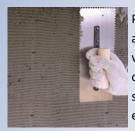
Place the veneer onto the adhesive and adjust to desired position, veneer should be firmly worked onto the substrate and pushed slightly back and forth to fully embed the veneer in the adhesive.
