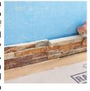
before you apply any adhesive, dry lay out your first row against the wall to help you work out the look you want. Lay them in a brick pattern to make panel joints less visible.
